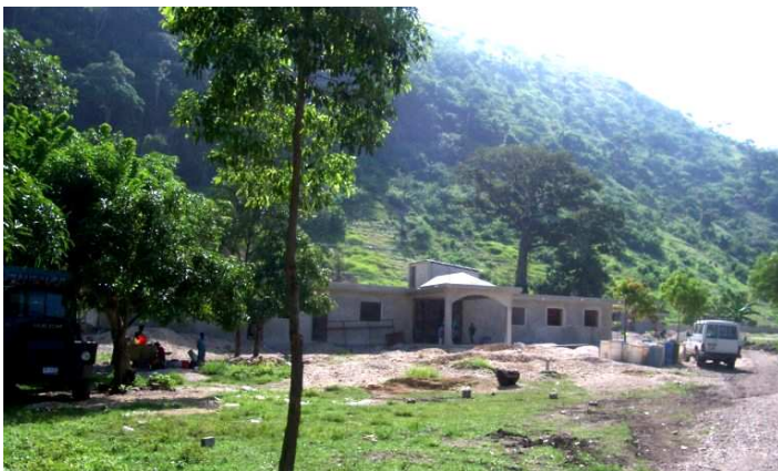
Progress is being made on the Lacolline hospital
