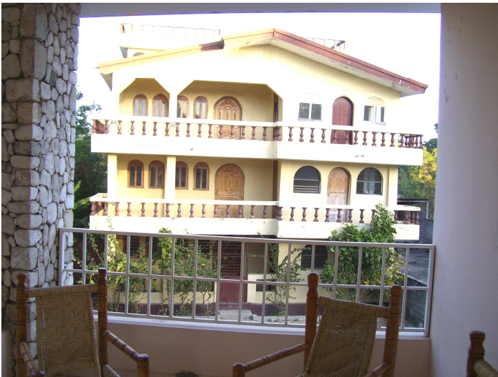
View of the girls' annex from the balcony of the administration building
